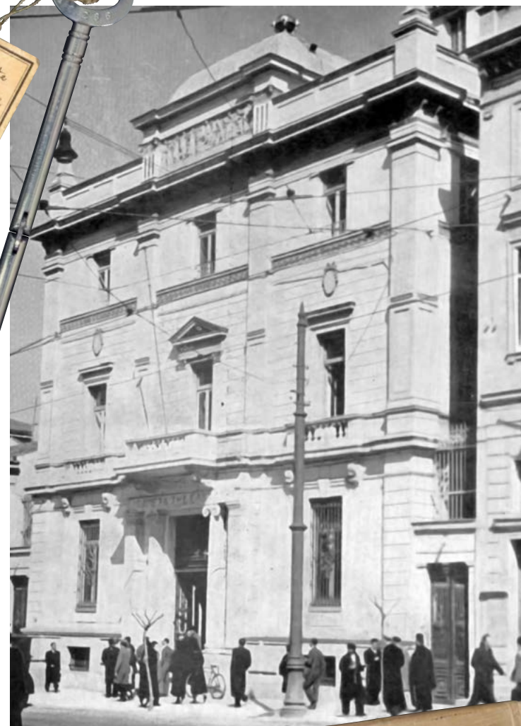
The key to the Simantiras mansion, where certain services of the Bank of Greece were housed in 1928.
